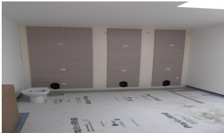
Toilet installation progress showing IPS panelling and sanitary works commencing
