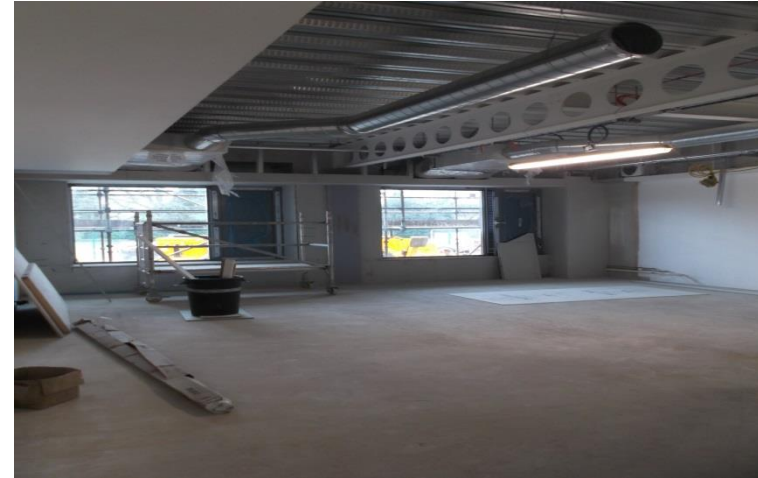
Typical classroom showing window progress
