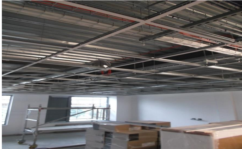
Suspended ceilings following bulkhead works
