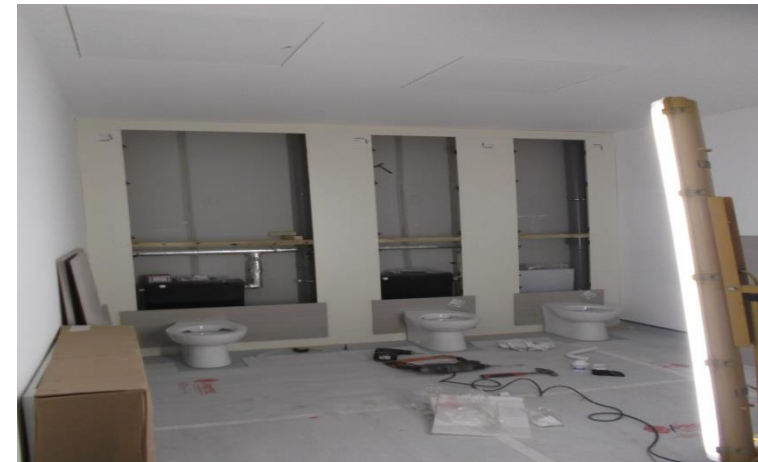
Toilet installation progress showing IPS panelling and sanitary works commencing
